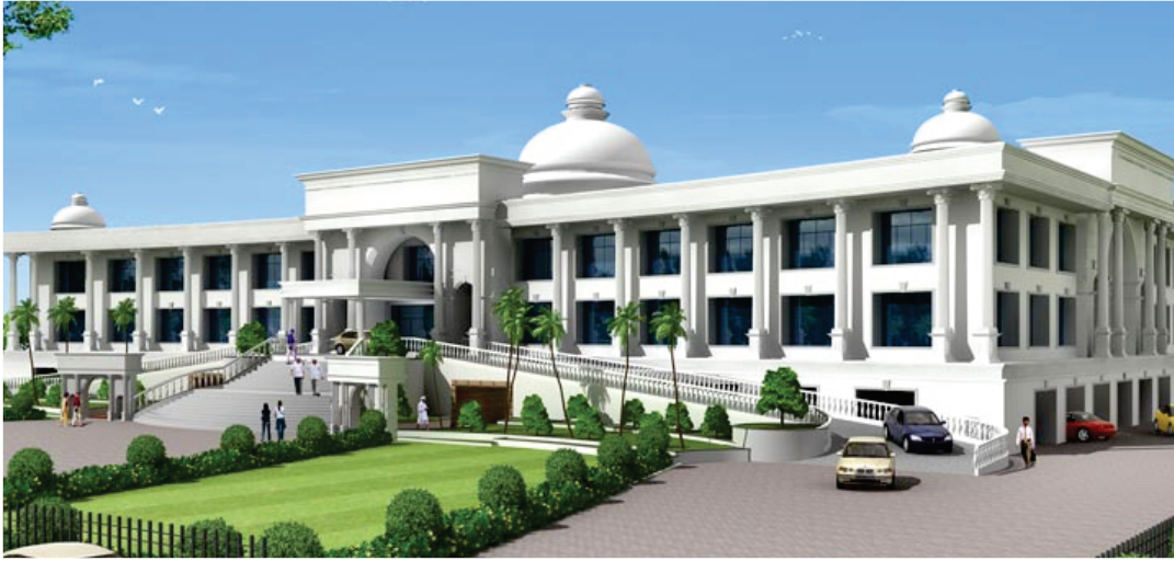
• New Collector office, Vishrambag.
